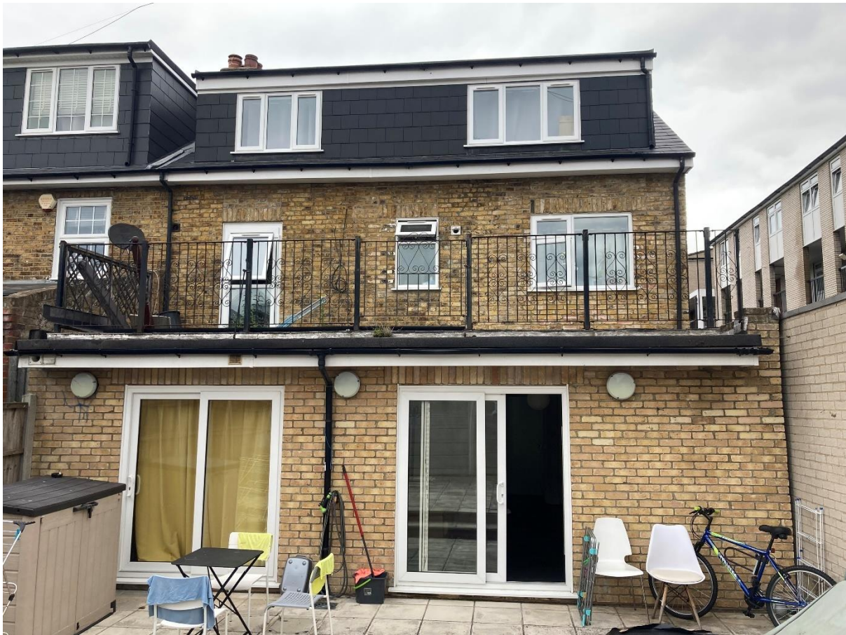
Rear view of the application property
